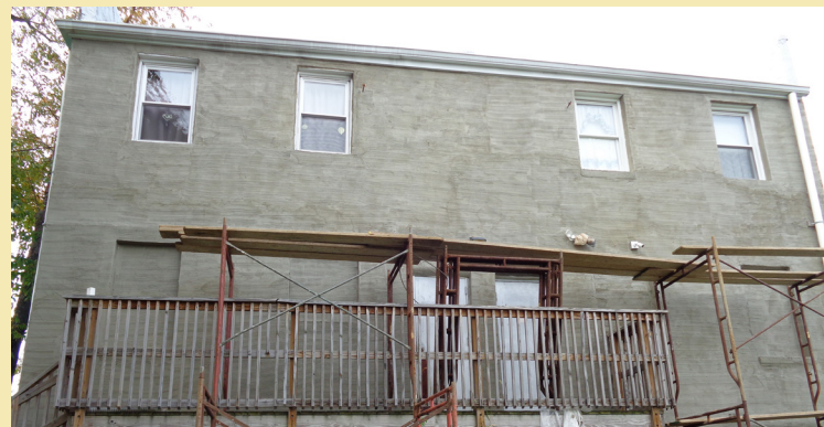
The back wall of the Bernardine Center underwent a major repair to prevent the rain from entering the building through large cracks in the exterior wall. We are grateful to W.W. Smith Charitable Trust for its grant.
